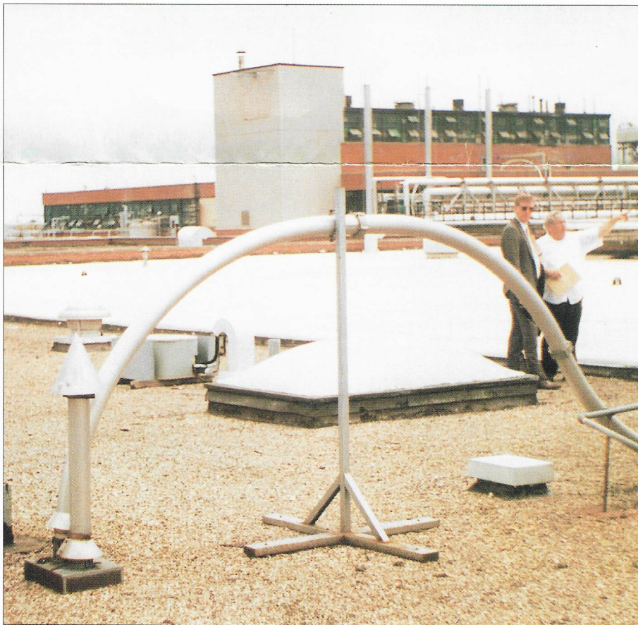
Pneumatic sample conveying system passes through roof over the lab and terminates in edible oil refining facility (background) approx 1050 ft away. Note that system draws air from outside building
